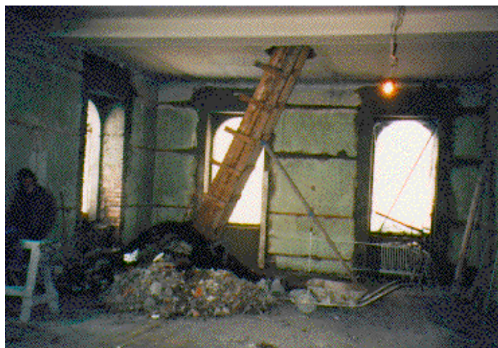
HNP Building Renovations
